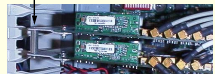
Standoff and Screw Installed
